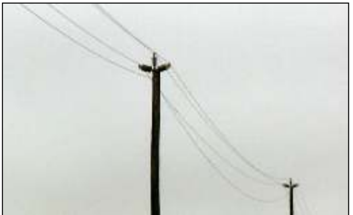
Above (a and b): Juvenile Osprey at the power line impact site Below: The Namdeb power line structures: 30kV "x-mas tree" configuration to waste management; in the background the 66kV line from ESKOM to the Namdeb substation.
