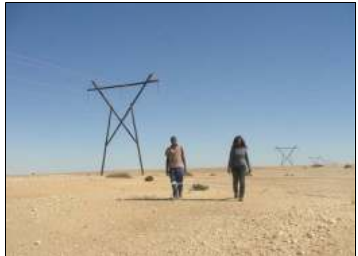
The Trekkopje-Wlotzka 132 kV line was surveyed on 24/8/11 by a dynamic team from Areva (Environment Management), including Kaarina Nkandi (right) and Richard Gurirab. This line is monitored regularly since the first flamingo collision incident was recorded here in July 2010 (photo: Areva).
