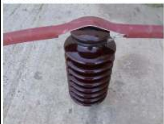
Step 1: Cut MVLC to fit over insulator head
