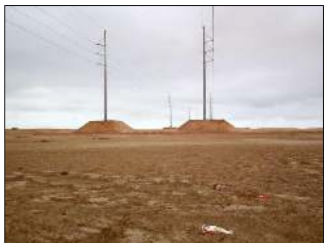
Flamingo collision (bottom right) on an unmarked section of the line (photo Ann Scott).
